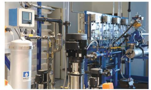
Pure Water Technology like microfiltration/ultrafiltration, reverse osmosis, and ultraviolet light/advanced oxidation are used to further treat recycled water to above drinking water standards. By the end of the decade, our region will receive 15% of its water supply from indirect potable reuse.
