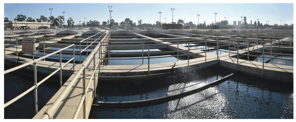
ocean. The demonstration facility purifies 500,000 gallons per day of the JWPCP's cleaned water using an innovative three-step process. First, membrane bioreactors remove ammonia along with other tiny particles. Next, molecules like salts are removed through reverse osmosis, which is the technology used for ocean water desalination. Finally, ultraviolet light and a powerful oxidant destroy
